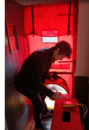
Airtight testing is a good baseline to look for leaks
