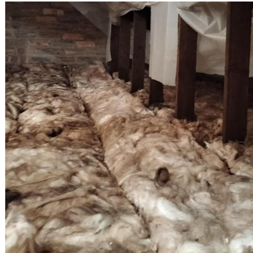
Insufficient and 'gappy' insulation on left and sufficient and continuous cover on right
