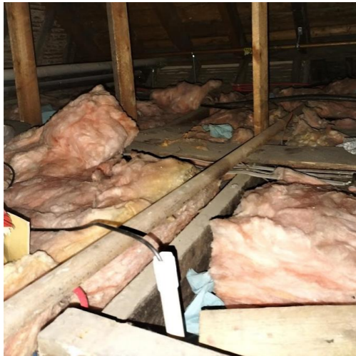
Insufficient and 'gappy' insulation on left and sufficient and continuous cover on right
