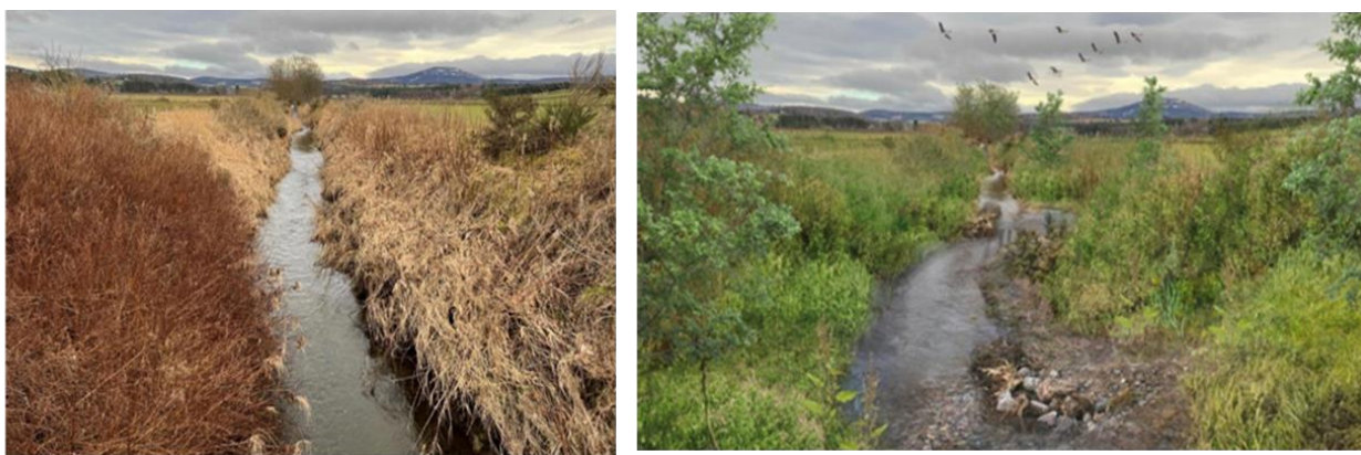
Figure 3-2: Example Channel Restoration through Large Woody Debris
